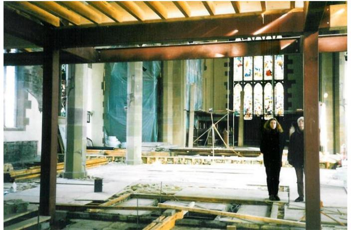
*Figure 11 - new steelwork goes in to support the balcony*
