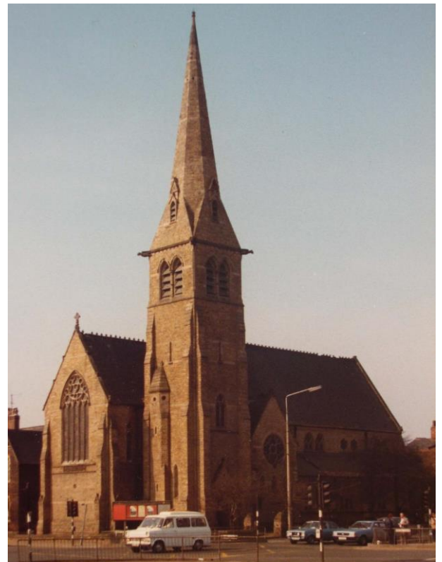
Stowell Memorial Church, Salford. Photographed shortly before its demolition.
